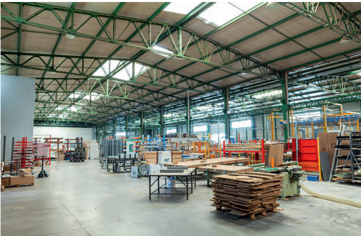
Stabilimento Mister Shut Establishment
